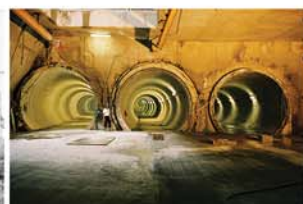
Tunel metrou Toulouse
